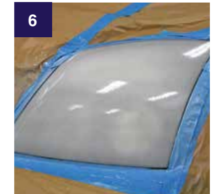
6 PRIMER APPLIED Primer appears dull / milky after drying.
