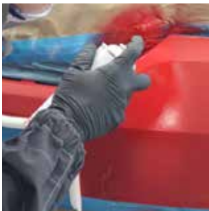
Apply basecoat to obtain adequate hiding.
