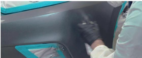
15. After performing a spray test, apply **Basecoat**
