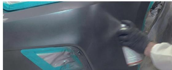
19. After activating **2K Clear Glamour 368-0061** and performing a test spray, apply over painted repair area
