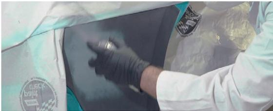
7. Apply a light coat of **Plastic Adhesion Promoter 368-0009** and allow to flash for 10 minutes before priming
