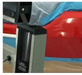
Damage: Scratched bumper. Use of an IR Lamp in between coats will aid in flash off (especially in high humidity conditions).
