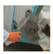
**Apply** 1 thin coat over repair area
