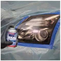
Apply a very thin (misty) layer of clearcoat first, directly followed by a continous, film-forming spray pass.
